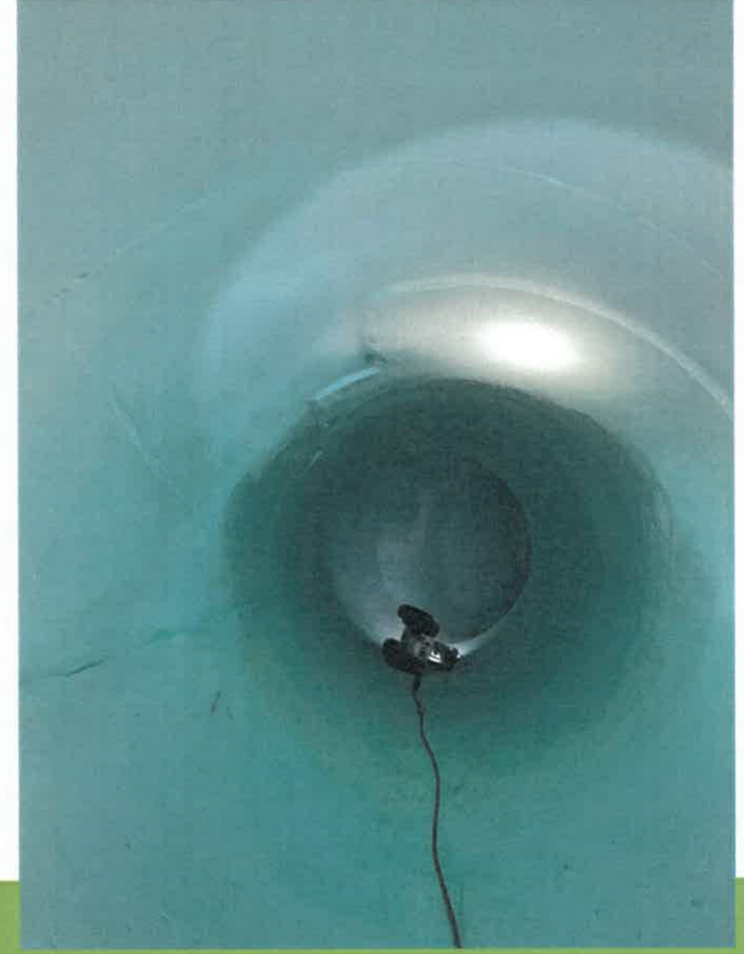
Cleaning/Prep of 66" Pipe & New Epoxy Lining
