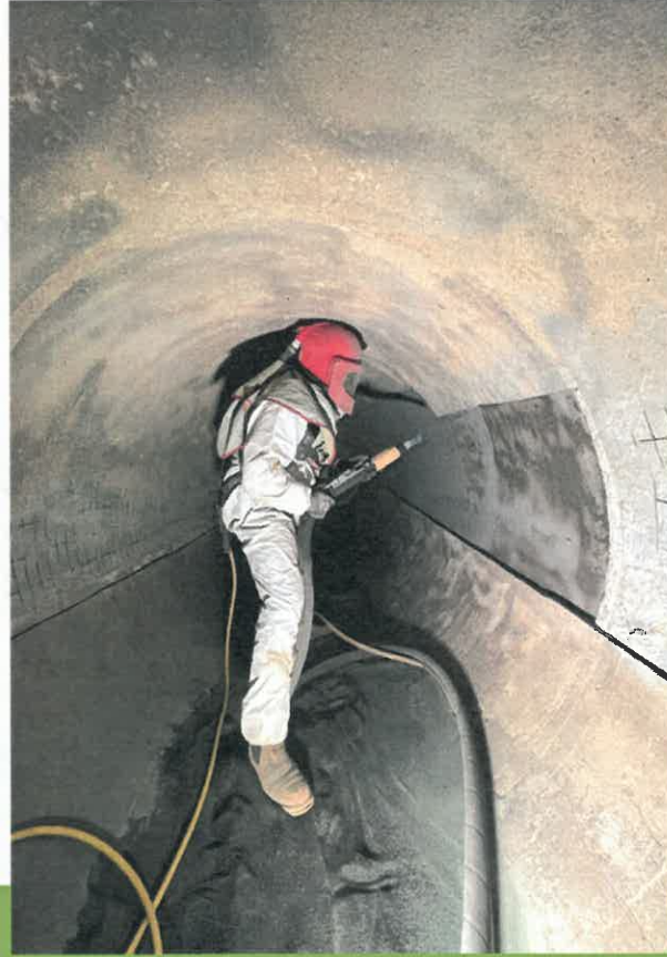
Cleaning/Prep of 66" Pipe & New Epoxy Lining
