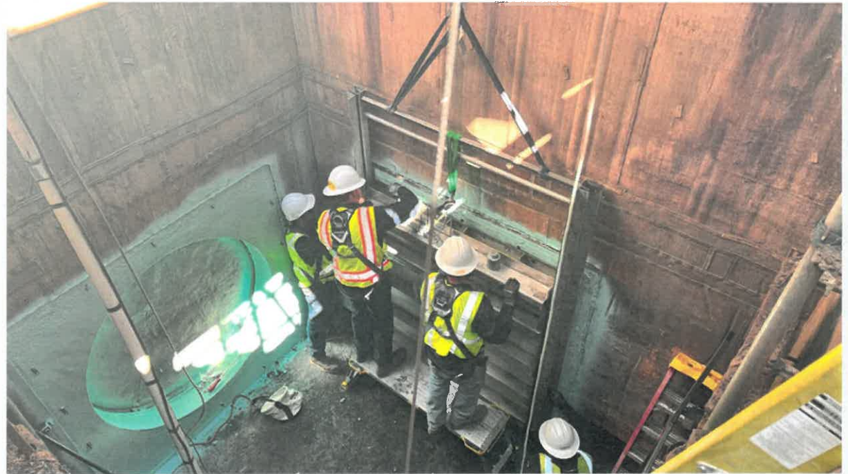
New Gate Installation in J-Box
